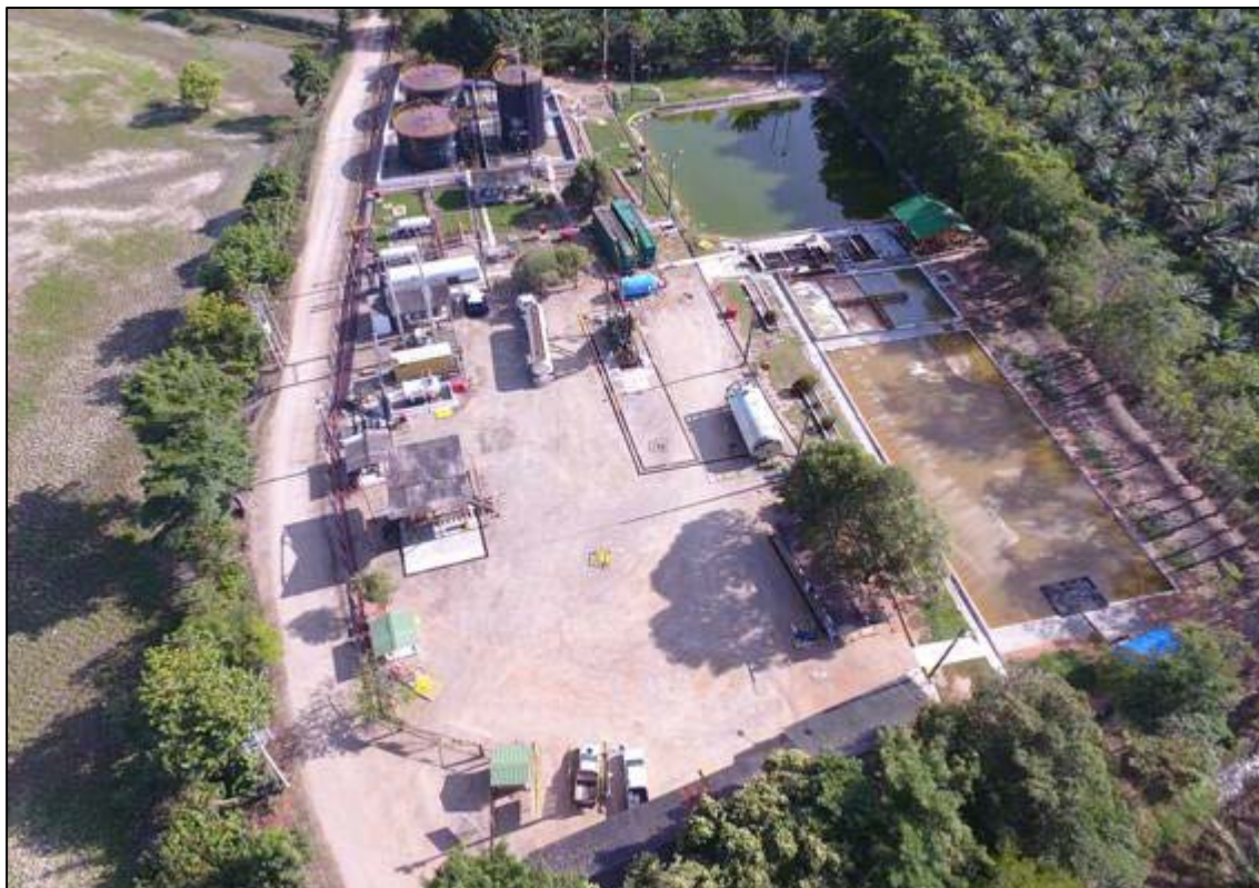
Figure 6: Aerial View of Santa Lucia Facility
