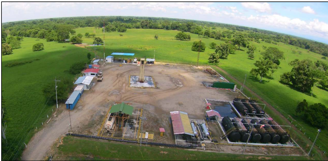
Figure 5: Aerial View of Colón Facility
